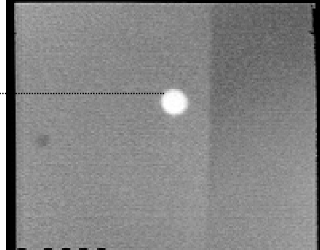
Thermal image of loose rivet
